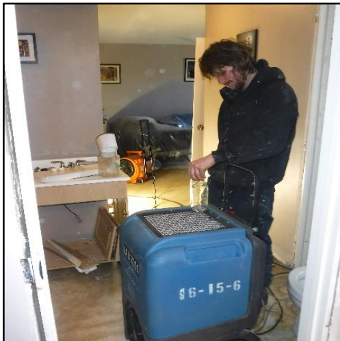
FLOODED SUITE: Dehumidifiers and fans must run 24 hours a day until the moisture is removed from the air
