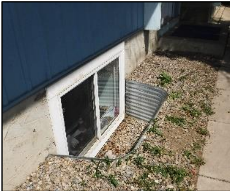
EGRESS WINDOW: Measured by the width and height of the open area
