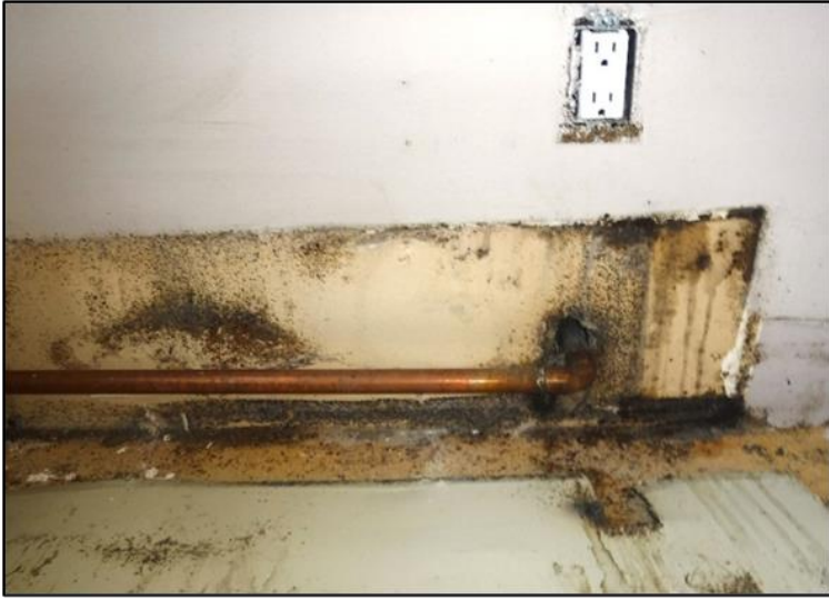
HEAT REGISTER: Thousands of bedbugs and eggs are found behind a heat register. Pest control poisons can't get behind heat registers and flooring or prevent bugs going in pipe holes
